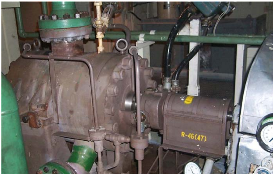
爐心隔離冷卻系統(RCIC)泵
