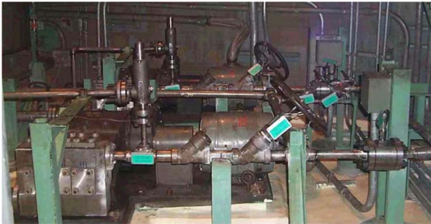
備用硼液系統(SBLC A/B)泵
